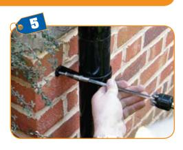
Fit the pipe clips to the downpipe and screw them into the wall.
