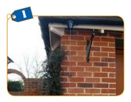
Using a plumb line, mark a vertical line on the wall from the outlet to the drain.
